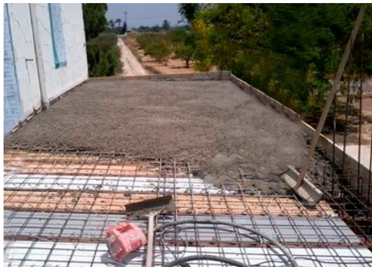
Figure 8.b. Rehabilitation. Concreting of the floor slab.
