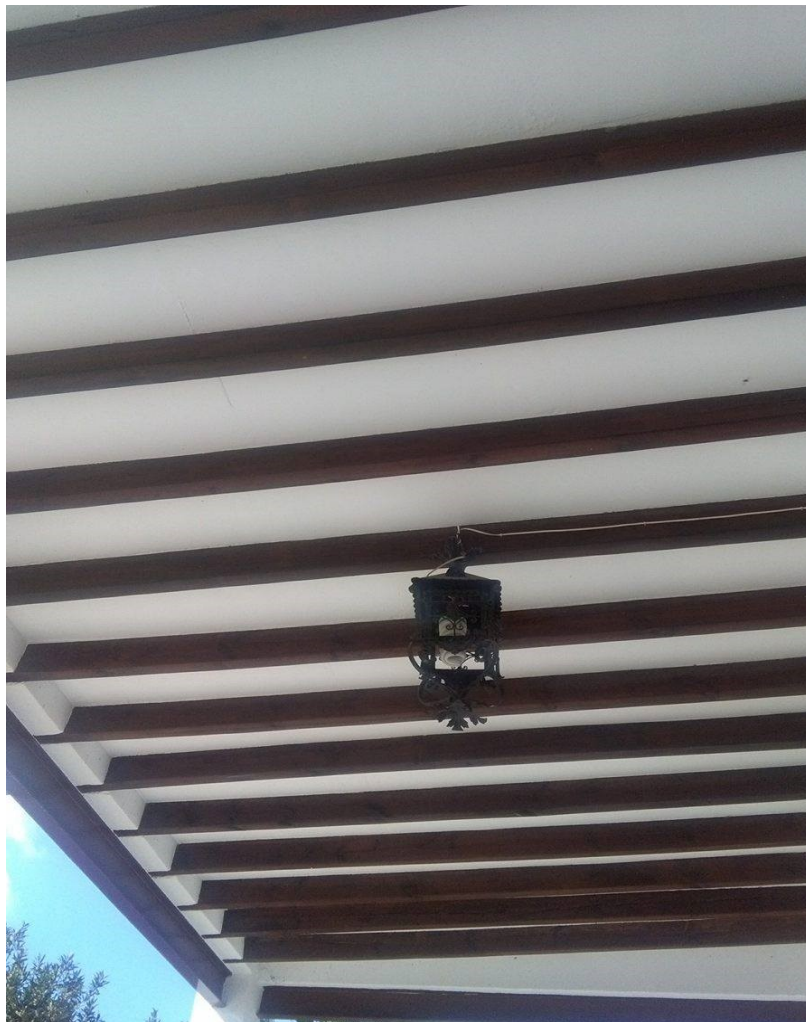
Figure 8.c. Rehabilitation completed, bottom view.
