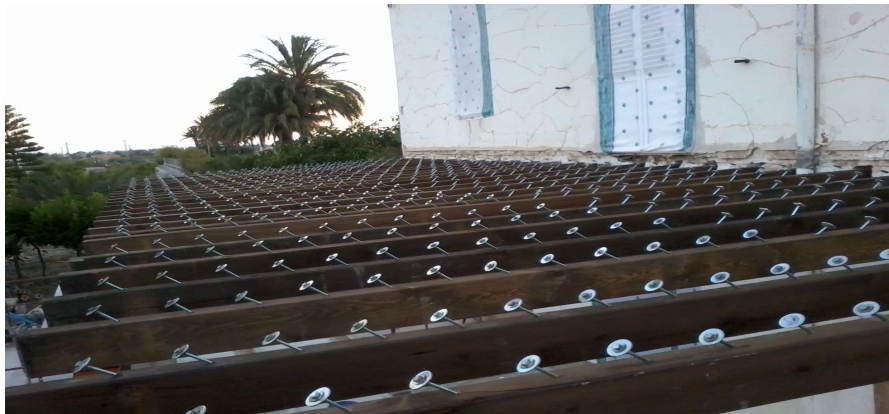
Figure 8.a. Rehabilitation. Beams with connectors.
