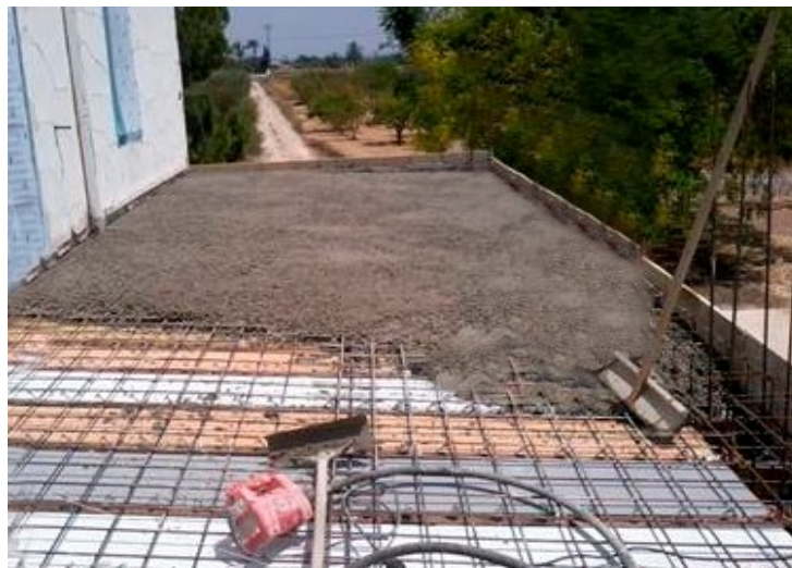
Figure 8.b. Rehabilitation. Concreting of the floor slab.
