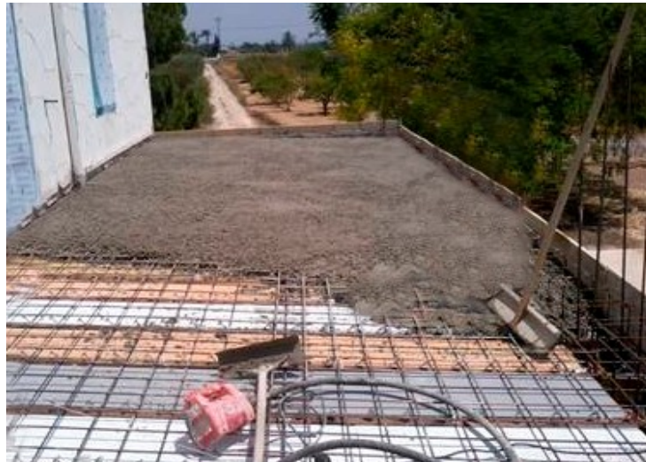
Figure 8.b. Rehabilitation. Concreting of the floor slab.
