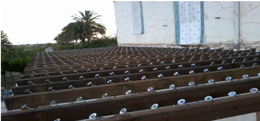
Figure 8.a. Rehabilitation. Beams with connectors.
