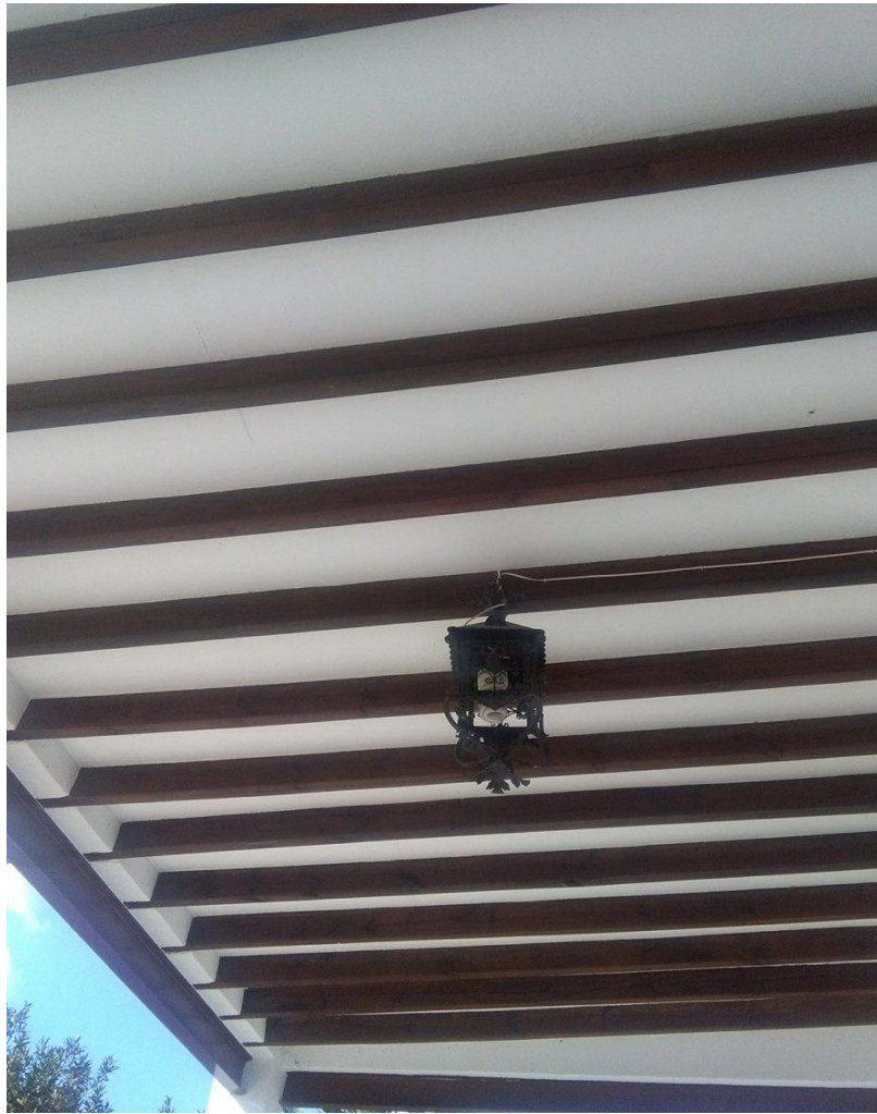
Figure 8.c. Rehabilitation completed, bottom view.
