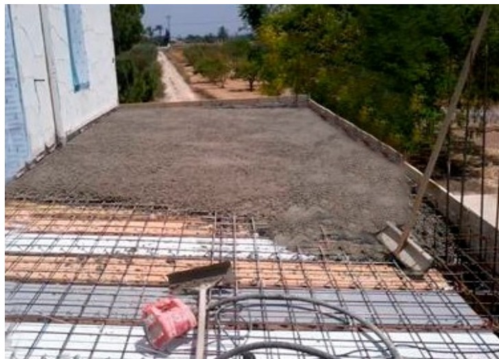
Figure 8.b. Rehabilitation. Concreting of the floor slab.
